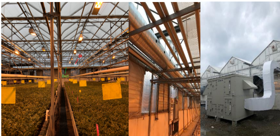
Figure 4 HRV and indoor ductwork in SA-5.
