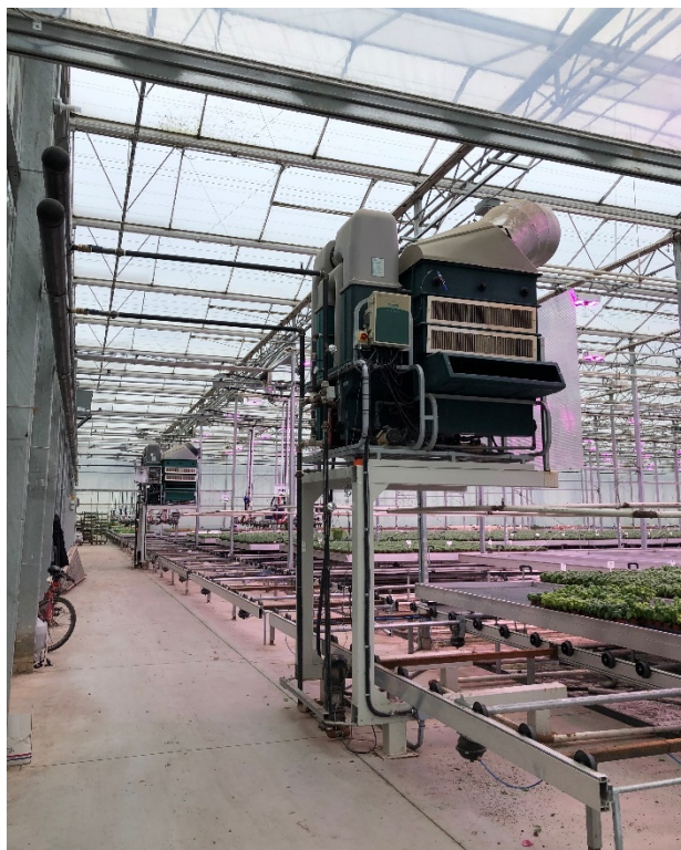
Figure 7 LDD units at SC-7 at the herb greenhouse.
