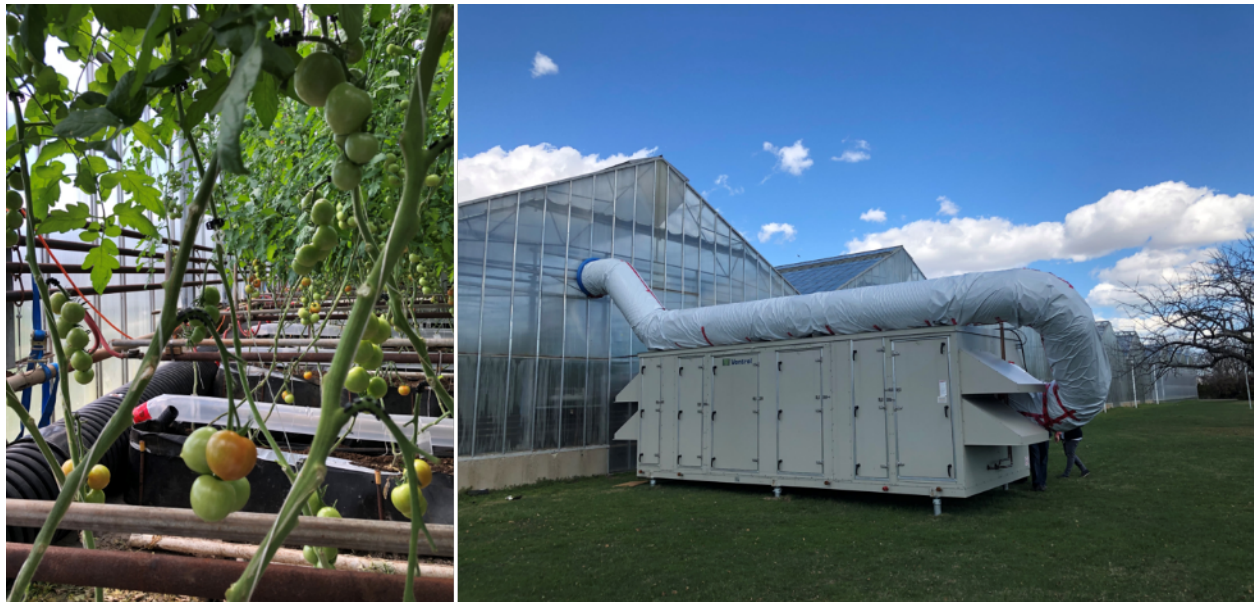
Figure 8 ERV and air ductwork at the vegetable greenhouse (Site D).
